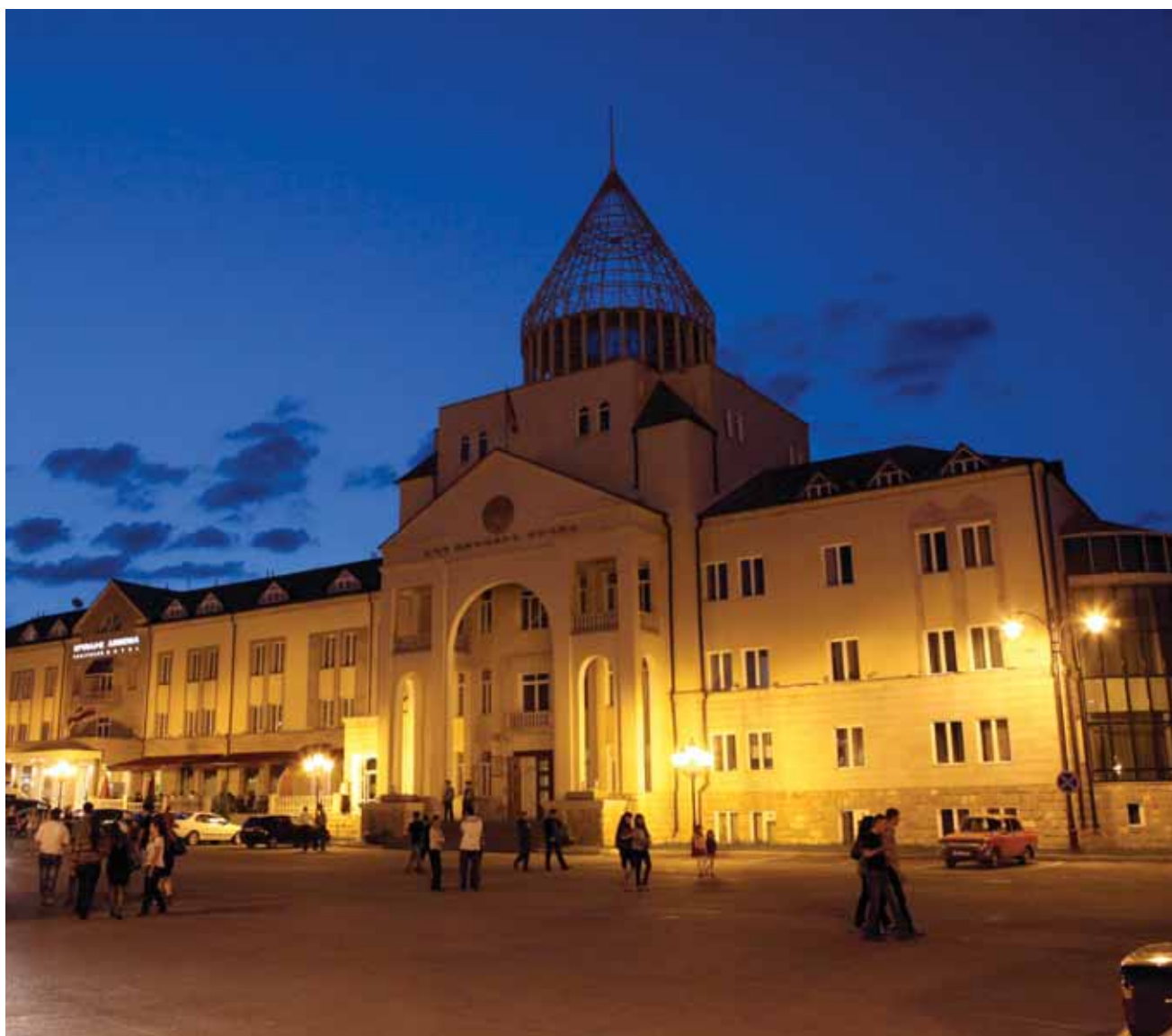
The MKR National Assembly building; Stepanakert, MKR.
